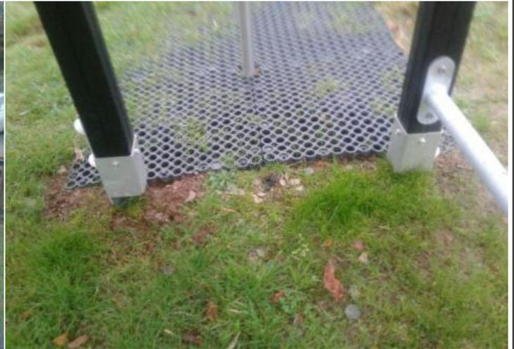
**Finding:** The edges of the grass mat surface have not been installed in accordance with the API Code of Practice
