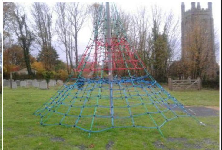
**Finding:** The connecting or tensioning ropes on the net are not tensioned correctly
