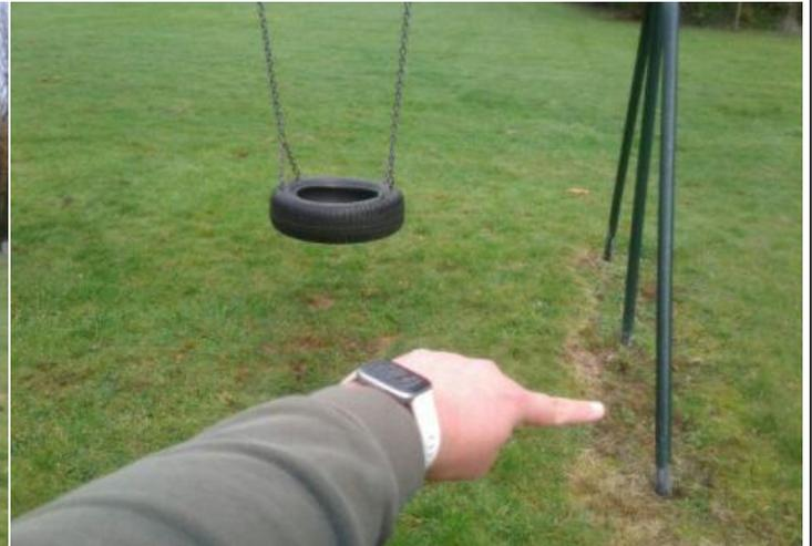
**Finding:** The surface has eroded and the foundations are exposed
