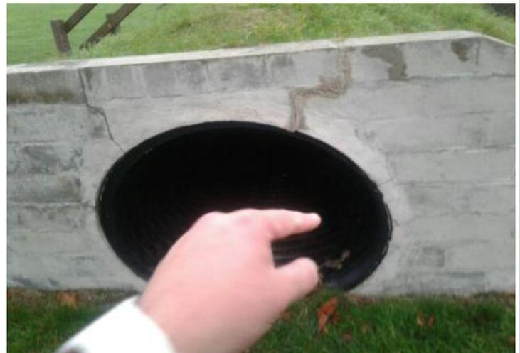
**Finding:** There are some rough edges of the plastic and concrete at the entrance on the tunnel
