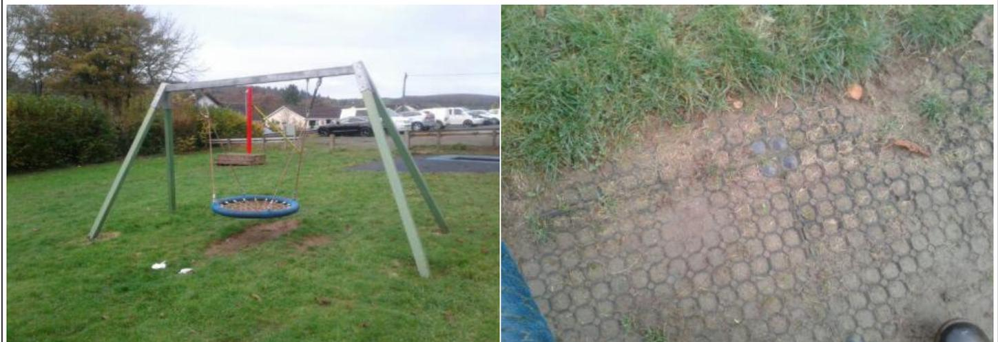
**Finding:** Fixing Pins have been installed in the impact areas of the grass mats
