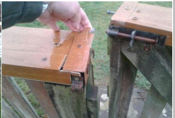
**Finding:** There is sharp sections of plastic on the fence next to the gate **Action:** Repair or replace
