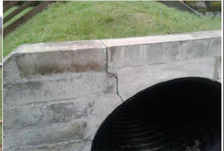
**Finding:** There are cracks in the wall
