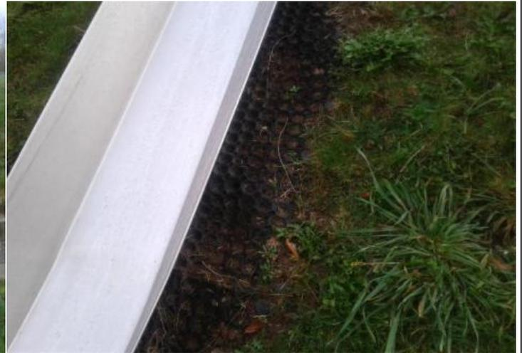
**Finding:** Fixing Pins have been installed in the impact areas of the grass mats
