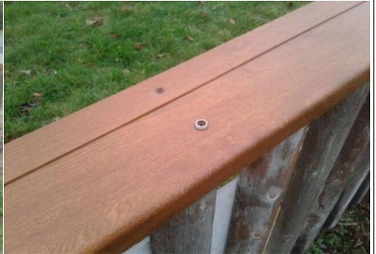
**Finding:** There is/are screw cap covers missing or damaged on the item **Action:** Monitor and replace if required
