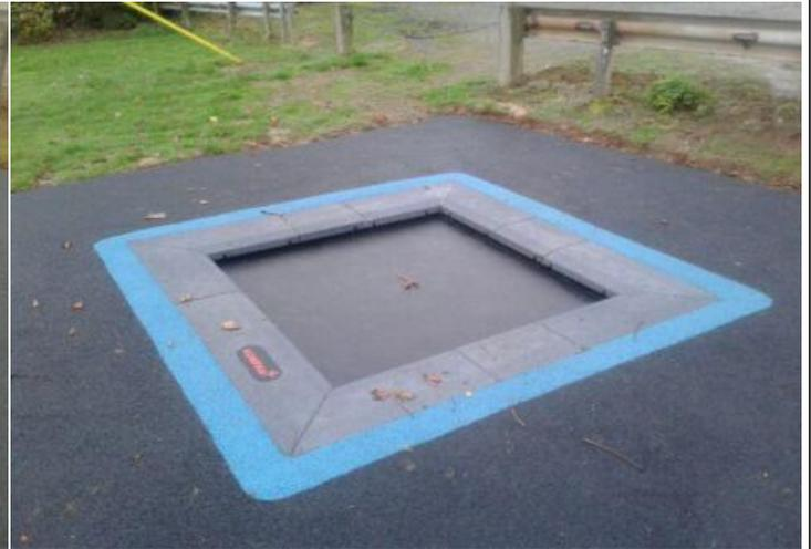
**Finding:** On site visits it is not possible to test the ground clearance of the Bouncing Facility bed as specified in BS EN 1176; ensure that the clearance between the Bouncing Facility Bed and the ground underneath is in accordance with the manufacturers recommendations (it was not possible to measure the depth at time of inspection measured unloaded due to the design of the bed of the bouncing facility).
