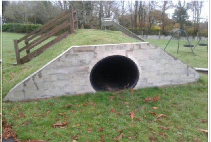
**Finding:** This design / configuration of tunnel mound is well established and has been successfully included in large quantities of playgrounds throughout the UK. Whilst the design does not fully meet the requirements of BS EN 1176 with regards to falls in excess of 600mm over the edge of the tunnel to the surface below, it has been risk assessed as fit for purpose and no changes are recommended to the design
